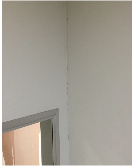
Fissura na parede do Home Officer
