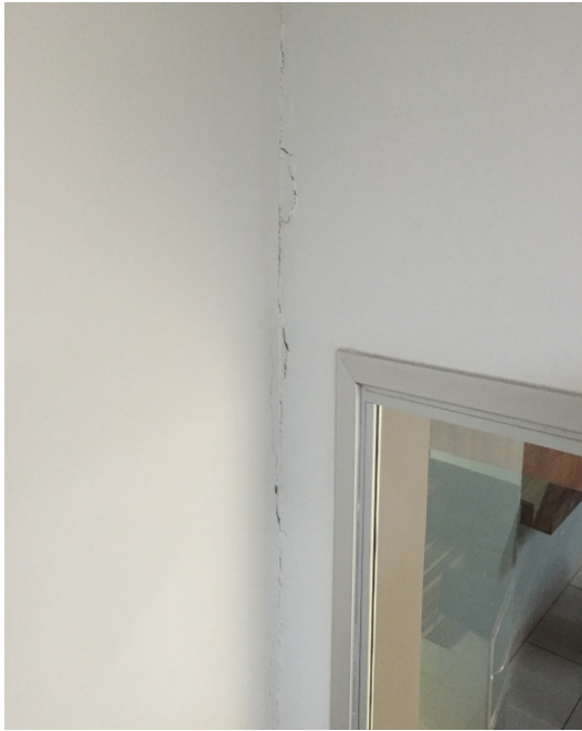
Fissura na parede do Home Officer
